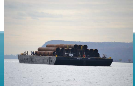
Piles mid-river en route to the New NY Bridge project.
