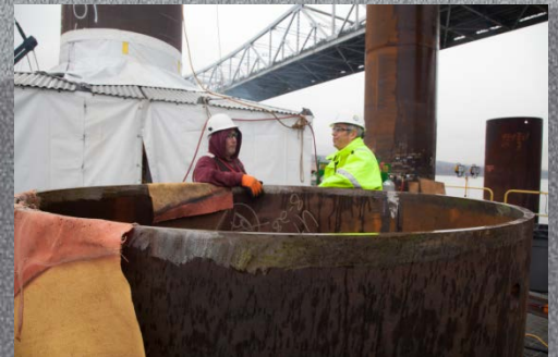
A 72-inch pile in place.
