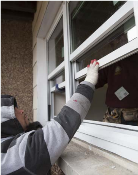
Installation of noise-reducing windows begins in Rockland County.
