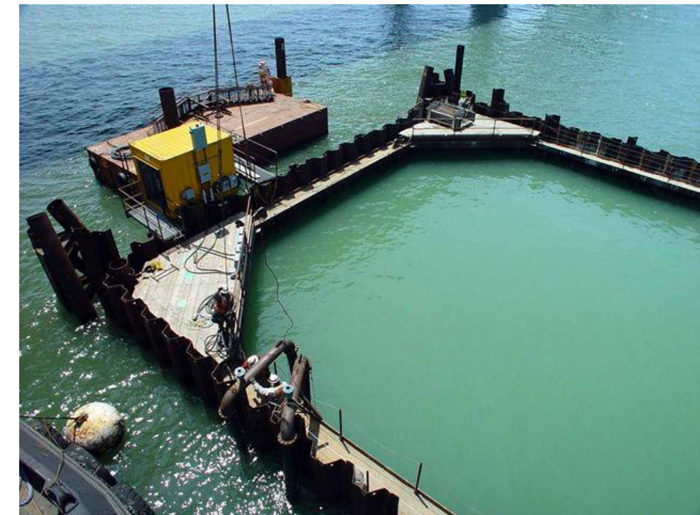
Figure 5-5 Cofferdams (Caltrans 2004)
